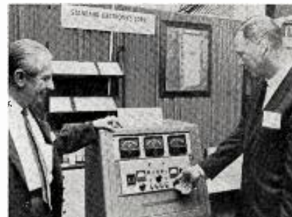
TV men must keep up with radio too. Chester Slaughter (r), WSPD-TV Toledo, Ohio, hears about new 250-w FM transmitter of Standard Electronics Corp. from Bill Stringfellow.
