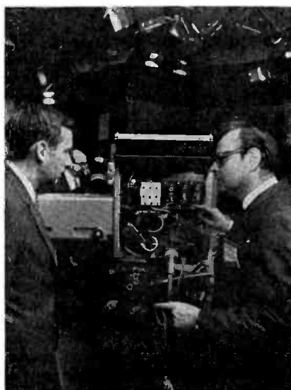
Latest version of the Norelco PC-70 Plumbicon color camera is given inside-out look for Frank Wheeler (l), KHON-TV Honolulu, by Abe Jacobowitz, broadcast sales manager, Philips Broadcast Equipment Corp.
