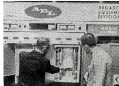
American Electronic Laboratories' Bill Bornmann (l) exhibits power tube details of 20 kw FM transmitter for Ron Toller, WEAM Arlington, Va.
